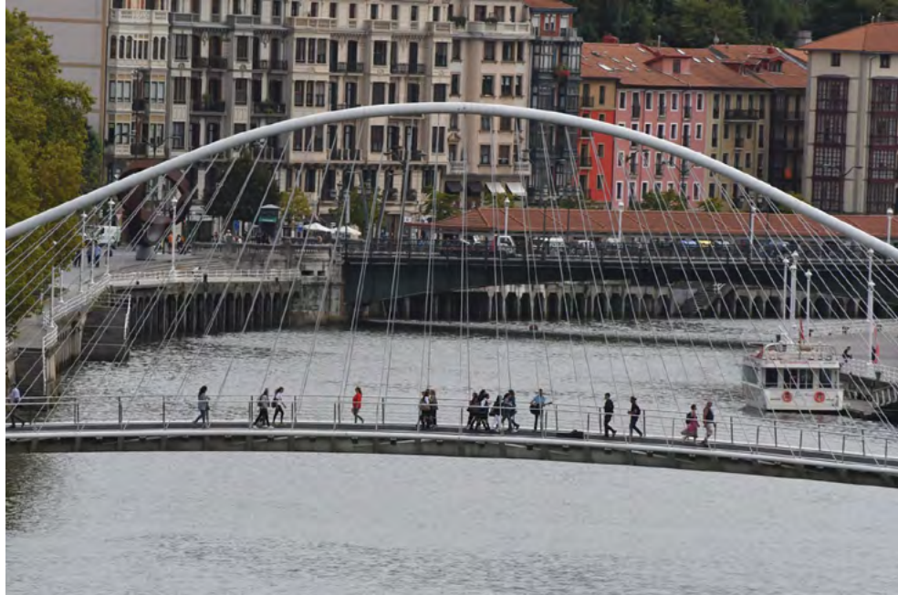
Puente Zubizuri, Bilbao Source: Bilbao City Council
