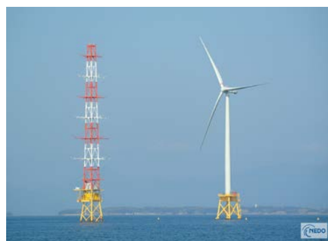
Wind power generation
