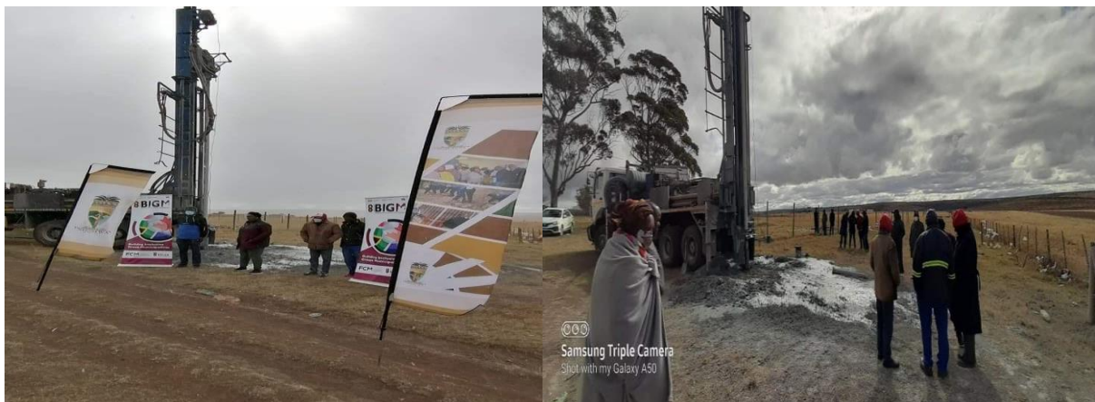
Figure 18: Drilling of Boreholes in Nqgushwa
