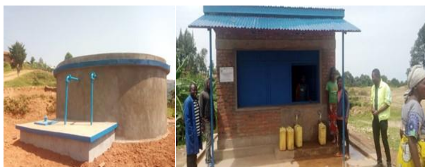
Figure 26: Rehabilitation and Extension of Rugobagoba-Tongati -Kizibaziba Water Supply System (68 km) in Karongi District
