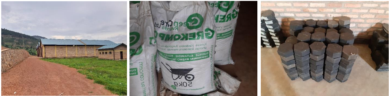
Figure 39: Huye district GreenCare Ltd youth run solid waste treatment in Sovu Industrial Park
