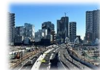
Loop road 2 (between Tsukiji and Shimbashi)
